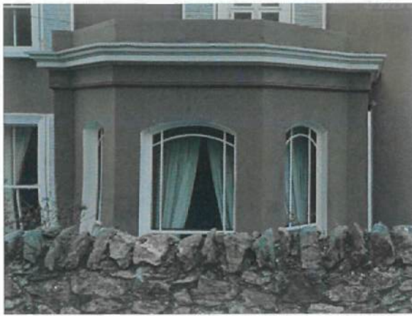
Changes to windows and cornice detail of projecting porch
